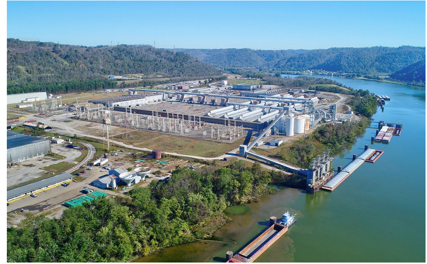
Long Ridge Energy Terminal
