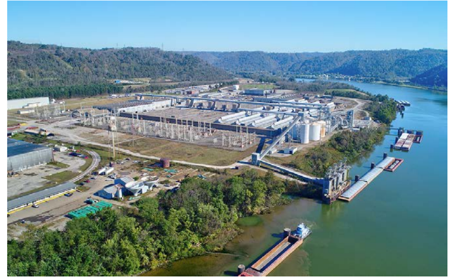
Long Ridge Energy Terminal
